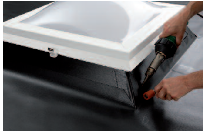
WOLFIN stainless steel sheets used for connecting rooflights
