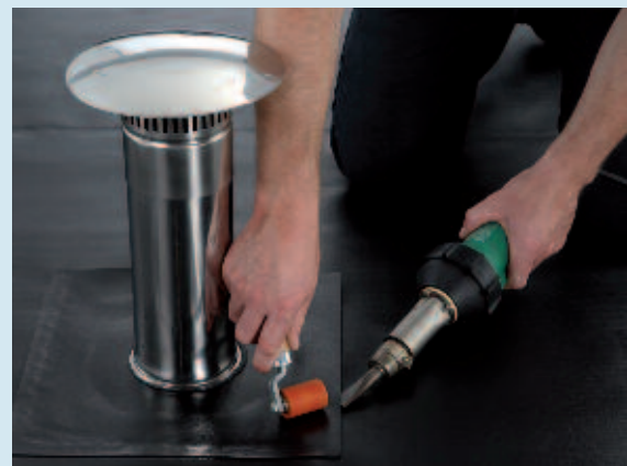
Connection to the adjacent membrane areas.
