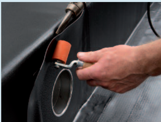
Connection of a membrane flange to the parapet
